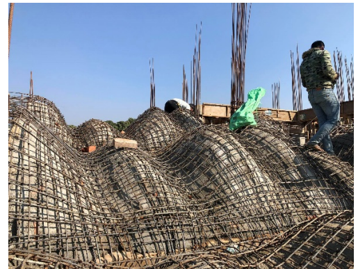
Figure 13. Reinforced concrete roof of a house, Nepal
