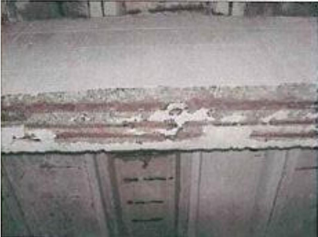
**Figure 1.** Corrosion of reinforcing bars in a beam
