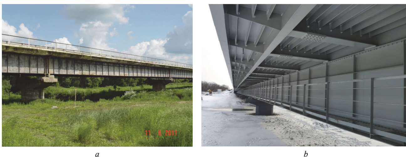
Figure 2. Side view of the span structure of the bridge across the Kabarga river: a – before overhaul; b – after overhaul, 2020
