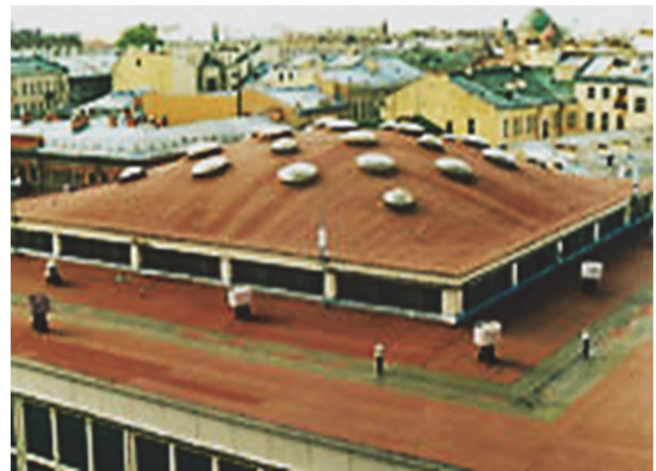
Figure 2. The gently sloping reinforced concrete pavement of the Nekrasovsky market in St. Petersburg, 1960 (Available from: www.g2p.ru)
