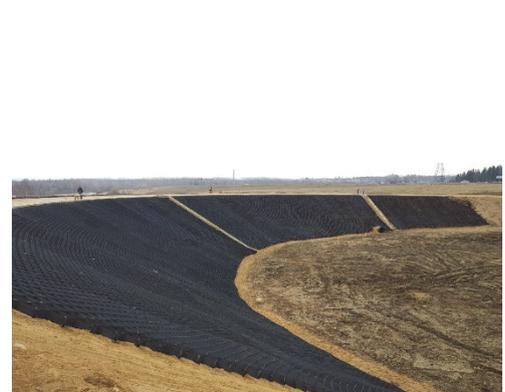
**Figure 9.** Strengthening of slope of the embankment when grade and rounding of the road (Available from: [https://www.geo-allianz.ru/objects/ukreplenie\\_otkosov\\_na\\_uchastke\\_dorogi\\_m-11/](https://www.geo-allianz.ru/objects/ukreplenie_otkosov_na_uchastke_dorogi_m-11/) (accessed: 30.04.2021))
