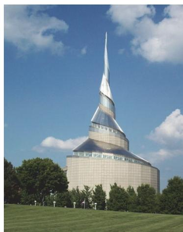
**Figure 5.** Torse covering in the form of a conical helicoid
