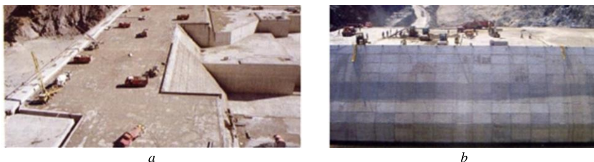
Figure 10. Top (a) and upstream (b) views of Cindere dam [20]
