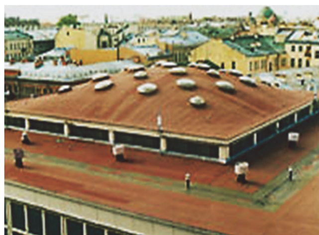
Figure 2. The gently sloping reinforced concrete pavement of the Nekrasovsky market in St. Petersburg, 1960 (Available from: www.g2p.ru)
