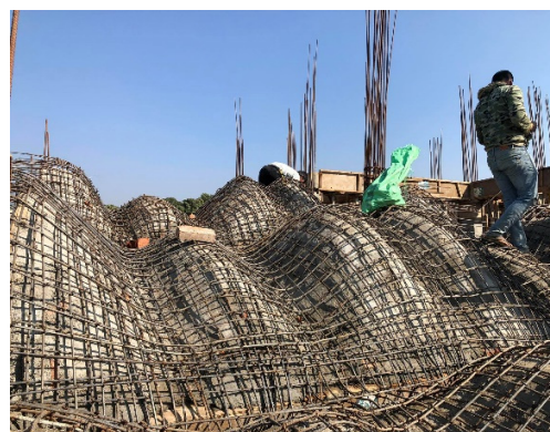
Figure 13. Reinforced concrete roof of a house, Nepal
