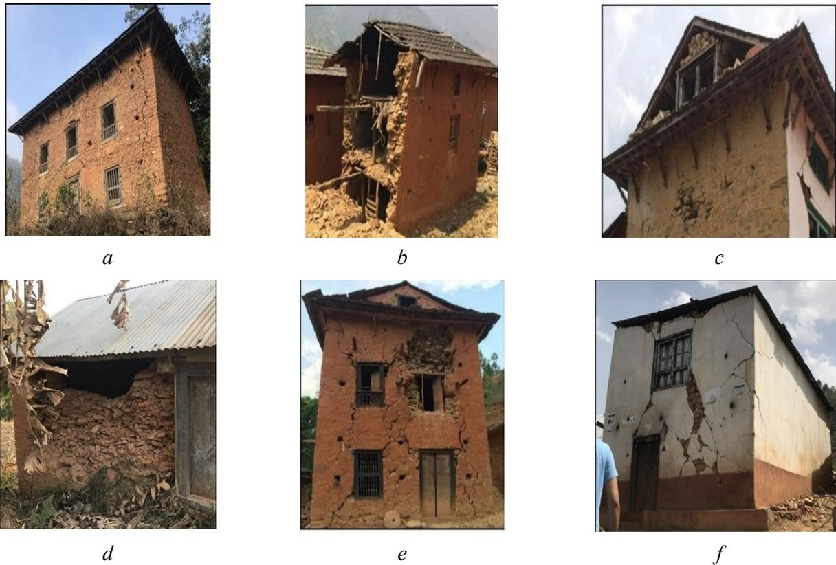
**Figure 1.** Failure mode in masonry building during earthquake:
