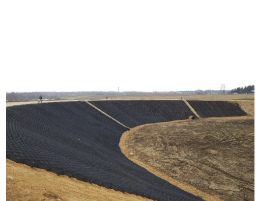
Figure 9. Strengthening of slope of the embankment when grade and rounding of the road (Available from: https://www.geo-allianz.ru/objects/ukreplenie_otkosov_na_uchastke_dorogi_m-11/ (accessed: 30.04.2021))
