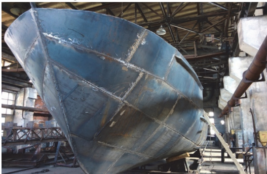
Figure 1. The erection of steel ship hull (Available from: ladverf.ru (accessed: 30.04.2021))
