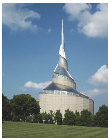
Figure 5. Torse covering in the form of a conical helioid (Available from: https://www.kcur.org/show/central-standard/2015-02-12/the-bloody-history-of-mormonism-in-jackson-county (accessed: 10.05.2021))
