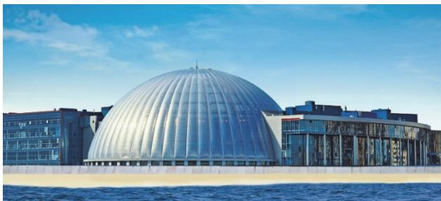
**Figure 7.** The biggest wooden dome in the world with a 43m height and a 90 m diameter, cultural-and-trade center “Piterland,” St. Petersburg, 2012
