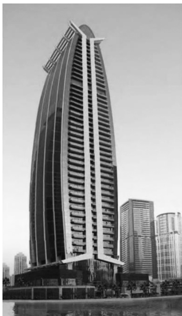
Fig. 3. Tiffani Tower, Dubai, UAE, 2010
